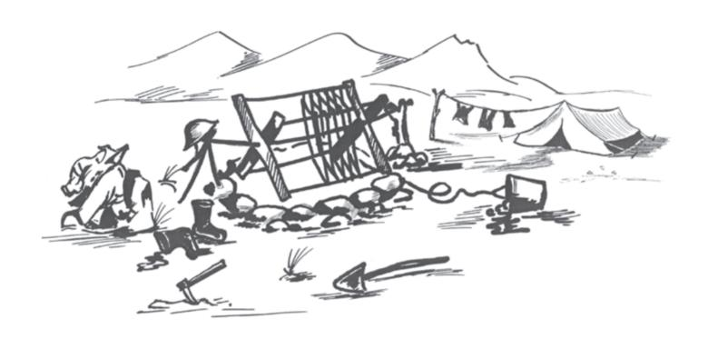
Daily attention should be paid to maintaining the above described work environment through renovation / rehabilitation process. Hence, at the end of each day, the well area should be cleaned of the excavated soil and silt; the rope on the wheel should be stored in place and the well exit point must be closed. The tools should be cleaned and stored in the shelter.
